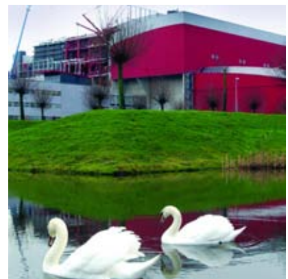
Alkmaar waste to energy plant, Netherlands
